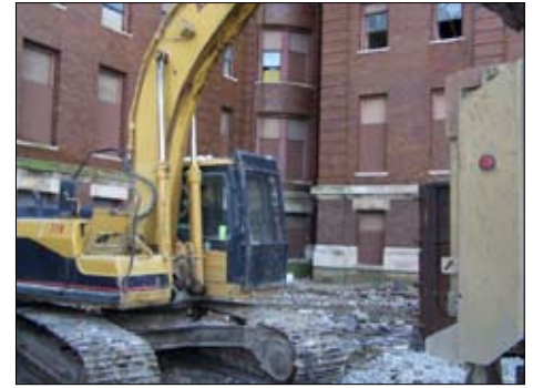
Doug Hubbard doing demo work at Ivy Tech in Indianapolis.
