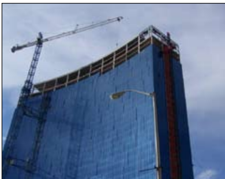
Kelli Seybold runs the tower crane while Tim Fields and Tim Browder run the hoist at the new Marriott in Indianapolis.
